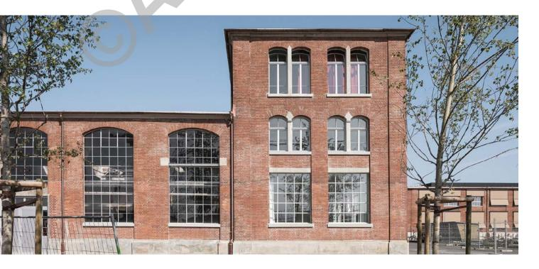
and then the roof and the façade underwent historically accurate renovation and restoration. The exposed brickwork of the eastern façade had to be cleaned several times by lye treatment.
